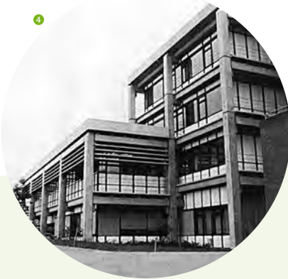
4 Exterior view of the Datacentre
